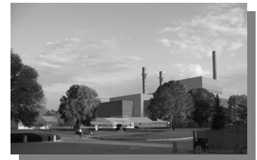
Proposed West Campus Cogeneration Facility
